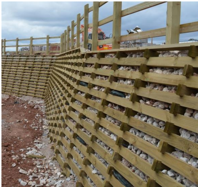
Figure 5 – Typical Permicrib Wall under construction
